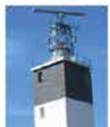
Coastal Surveillance System
